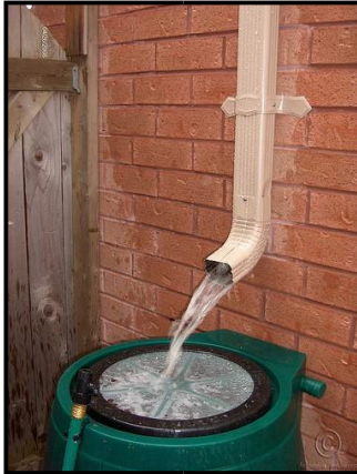
Figure. 4 Rainwater collection (through downpipes and sieves)
